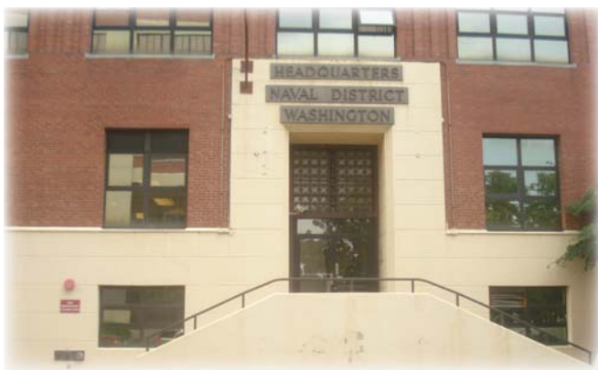
Washington Navy Yard B200 Five-Story Building Exterior
